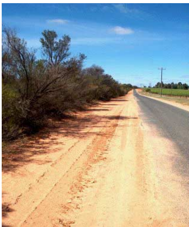
Fig. 3. Murraylink, after cable installation
