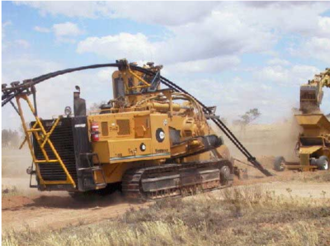
Fig. 6, Vermeer Trench excavator in action
